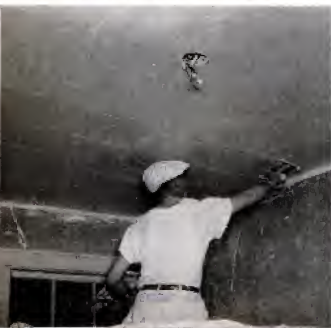
Ready-mixed plaster is applied in thickness of 1/16 to 1/8 in. and good workability permits long, sweeping strokes with trowel, as shown in the photo below
